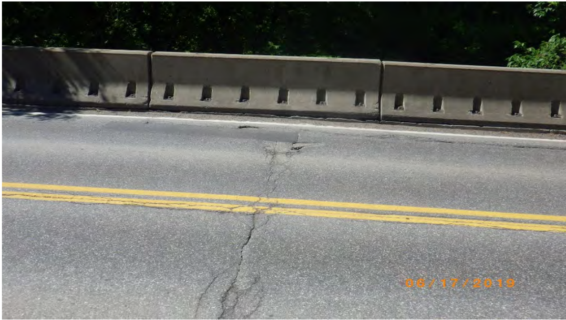
Picture 5: Concrete Barrier Railing
