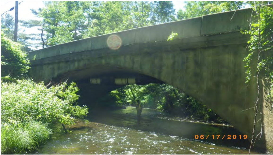
Picture 7: Upstream Fascia
