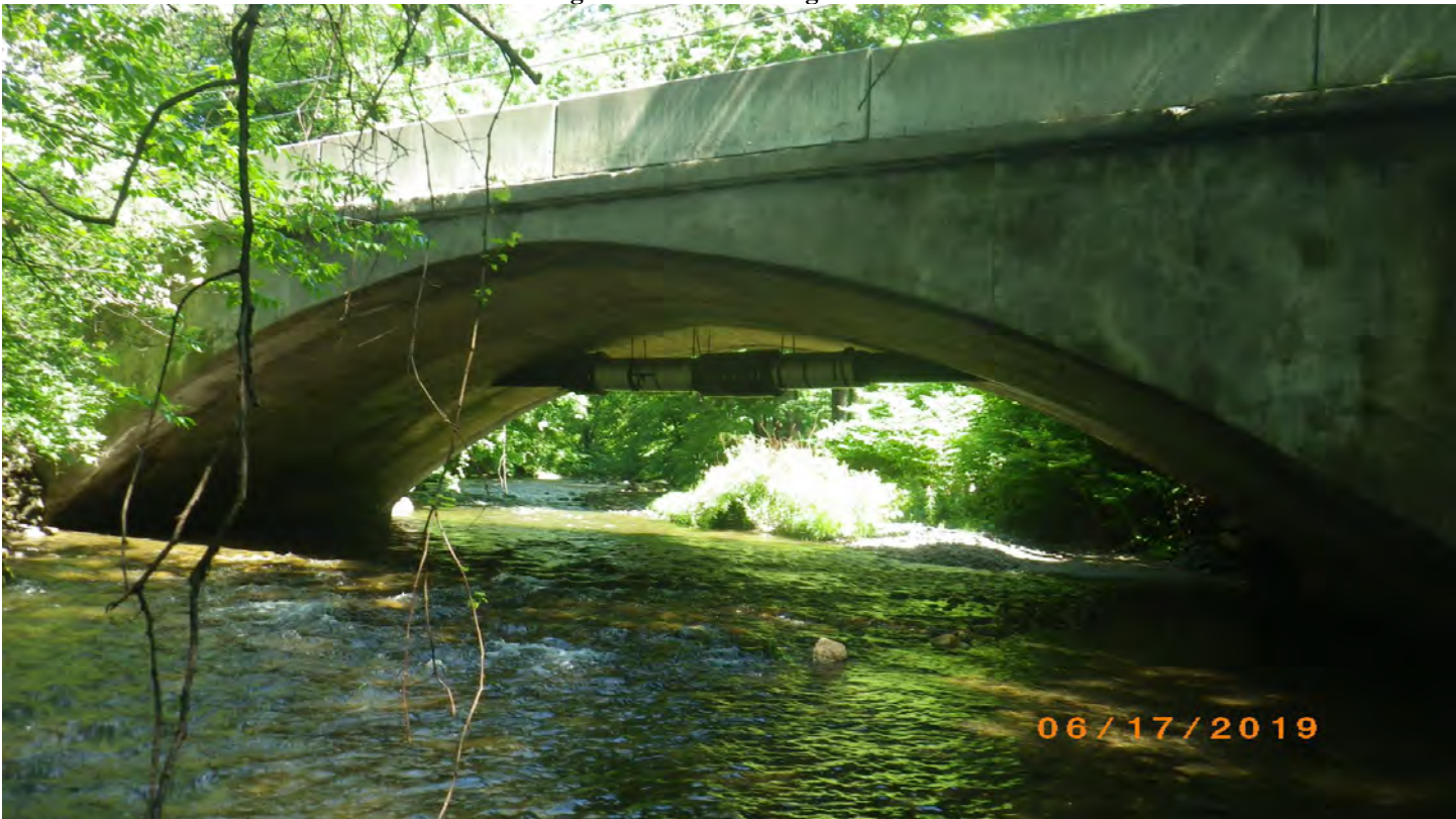
Figure 6: View of Bridge North.
