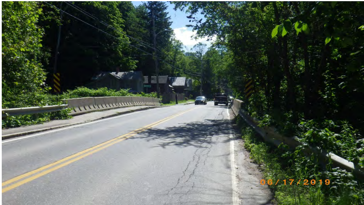
Figure 3.1 Looking eastbound on VT Route 9; notice overhead utilities present running parallel to westbound travel lane. [Inspection photo dated 2019].
