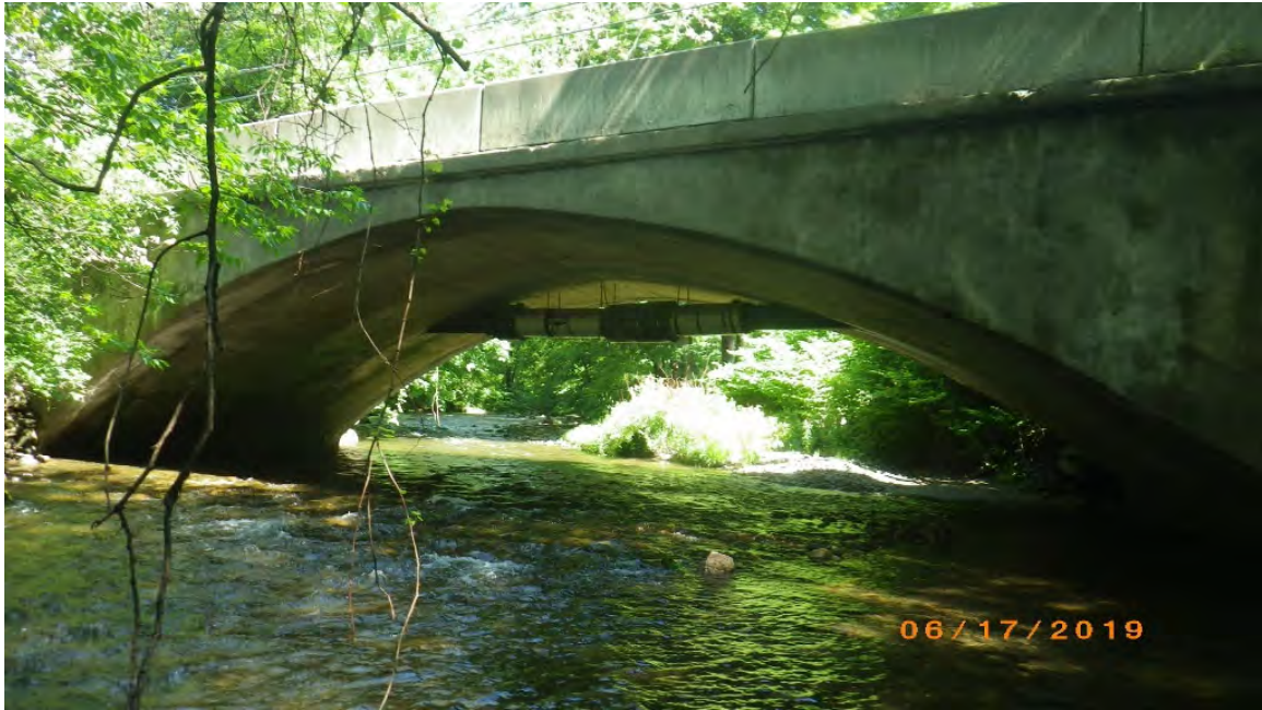
Picture 8: Downstream Fascia
