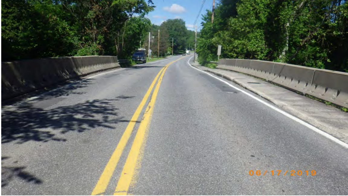
Picture 2: Looking West over Bridge 54
