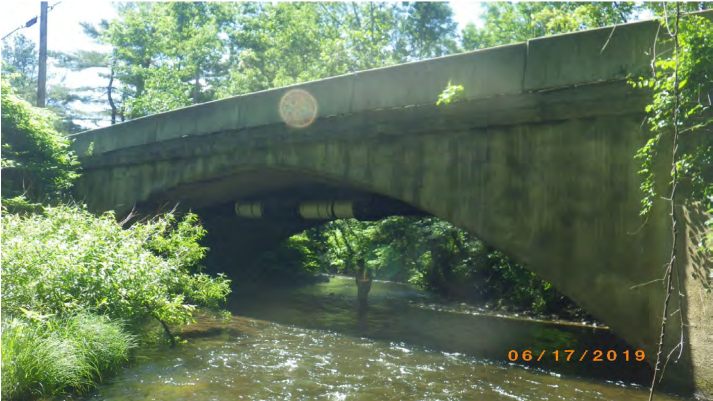
Figure 5: View of Bridge South.
