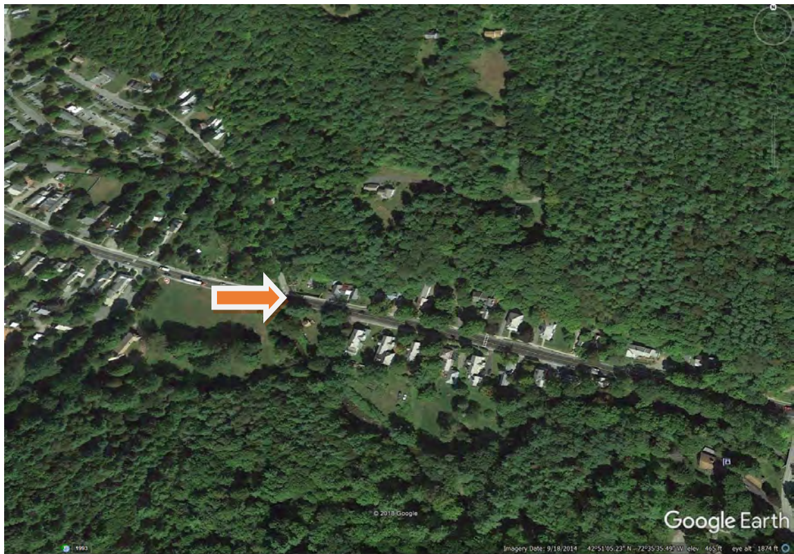
Figure 2: Aerial View of Project Area.
