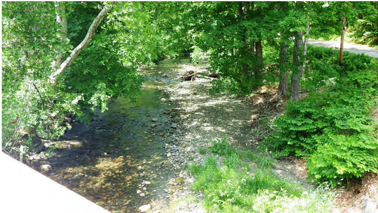
Figure 3.2 Looking upstream of Whetstone Brook; notice cobbles in the streambed. [Inspection photo dated 2015]
